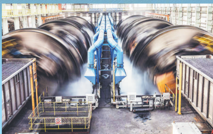
黄骅港三期翻车机房。梁雪冰 摄
